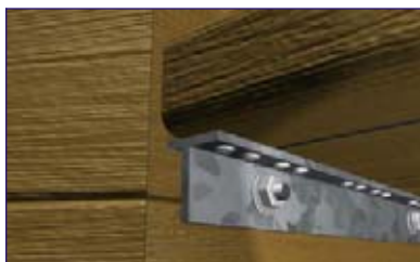
Assembly by means of T-profile and nuts
